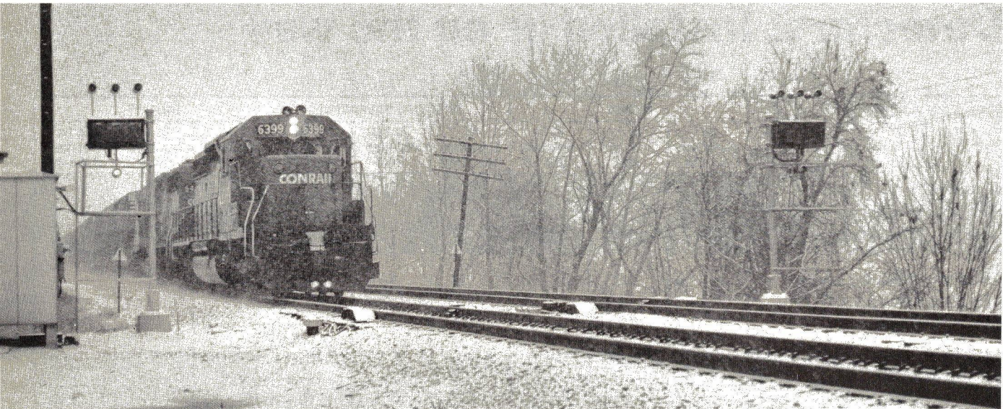
Conrail hot box detector installation at Harmersville, Pa. with display board readouts. Following highly favorable train crew reactions to its first 11 "talker" installations in 1980-81, Conrail began large-scale applications and currently has more than 450 hot box, hot wheel and dragging equipment detectors with voice readouts, generally providing more complete information on multiple detectors than practical with the limited number of auxiliary indication lights used along with the axle-count display board.
